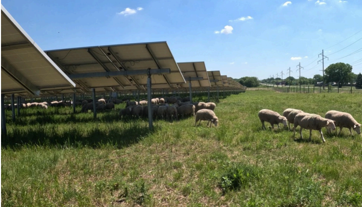
Sheep grazing under solar panels. Credit: University of Minnesota
